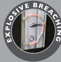
Cutting charge on head locks
